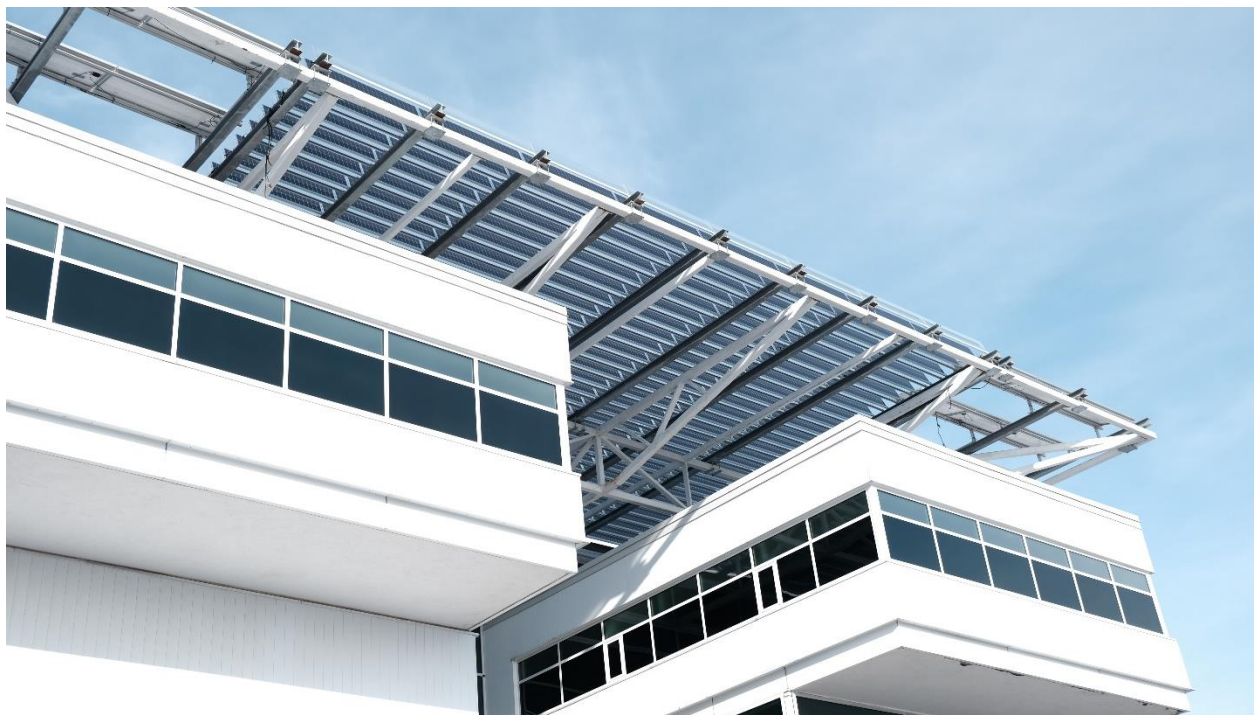
SPOTlight Solar Pergola at OAA headquarters seen from street level.
